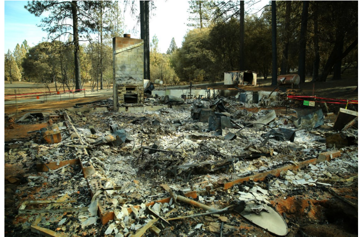
The 2015 Butte fire in California scorched 110 square miles of public and private property, including this single-family home. Over 549 homes were burned down to the ground as a result of fast-moving wildfires that were catastrophic to this community. Photo by Adam DuBrowa/FEMA
