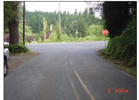
Northbound Slick Rock Road Approach
